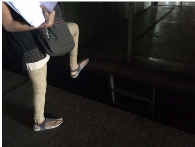
Figure 6: Platform-footboard gap on platform 1
