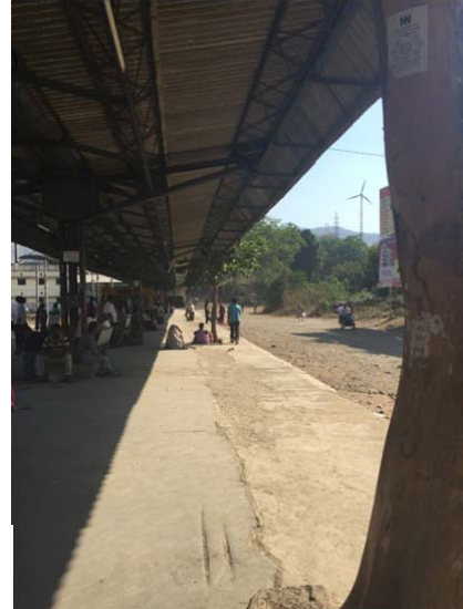
Figure 11: Figure 10: Entry Exit Point at Khopoli Station
